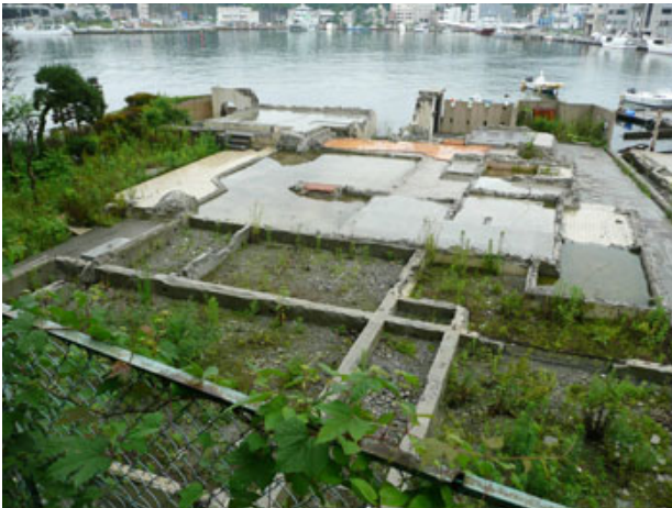
“A Foundation For What Used to Be A House”
